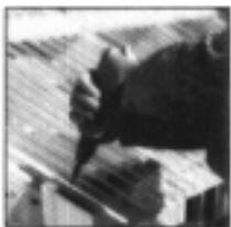
Drill with a high-speed steel- or carbide-tipped twist drill. Drill holes slightly larger than the fastener to allow for expansion and contraction (e.g., drill a 1/4" hole for a 3/16" screw). Place holes at twice the fastener diameter or 1/2" from the edge of the sheet, whichever is greater.
